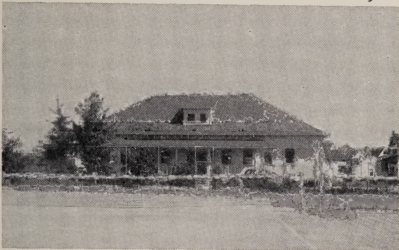
Agnes L. Park Recreation Building — Dedicated July 8, 1949
